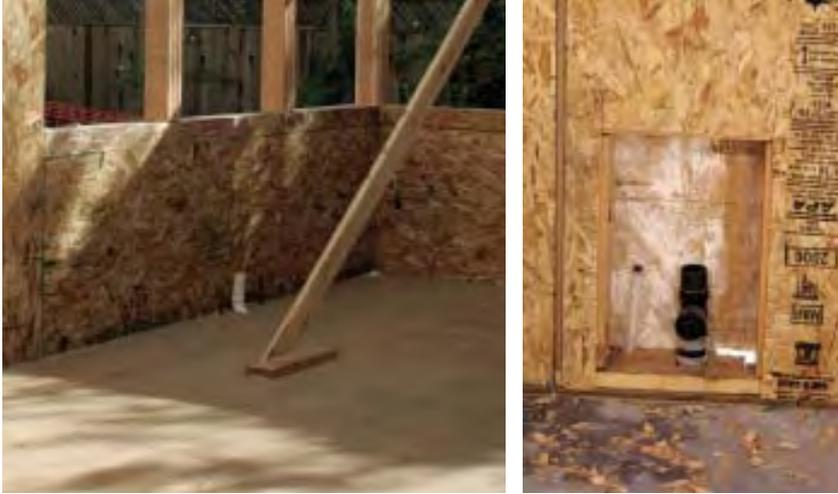
**Figure 10.** To avoid putting pipes in the wall, the author had the plumber install the drain and supply lines for a sink just inside the panels at the sink-cabinet location (far left). If plumbing must go in an exterior wall, the author creates a chase by cutting out the panel and removing some of the foam (left). Once rough-in is complete, the author's crew uses spray foam to fill in around the pipes.
